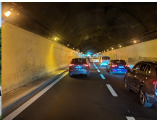
Tunnel in Bolzano -
